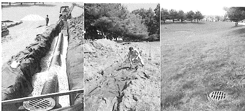
Figure 4: Example of Infiltration Trench Installation
