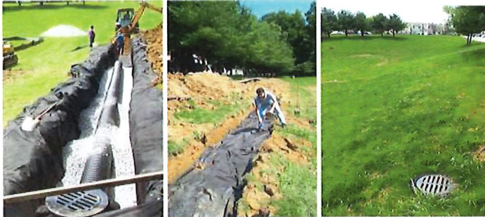
Figure 4: Example of Infiltration Trench Installation
