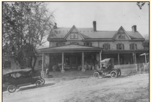
Holland general store around 1915. Note that the level of Buck Road has been raised by this time and the horse-drawn carriage has been replaced with the automobile.
