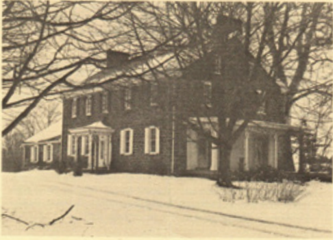
MAIN HOUSE, LOOKING SOUTH
