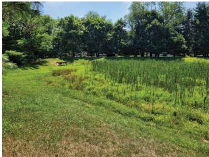
JENNIFER LANE BASIN OUTLET STRUCTURE
