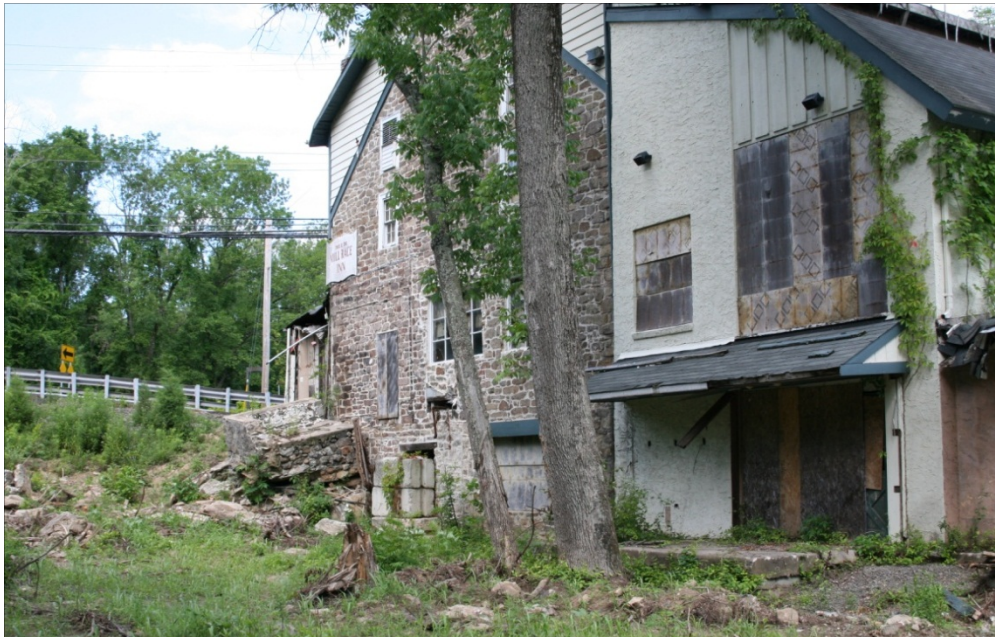
Mill Race Inn, south façade.
