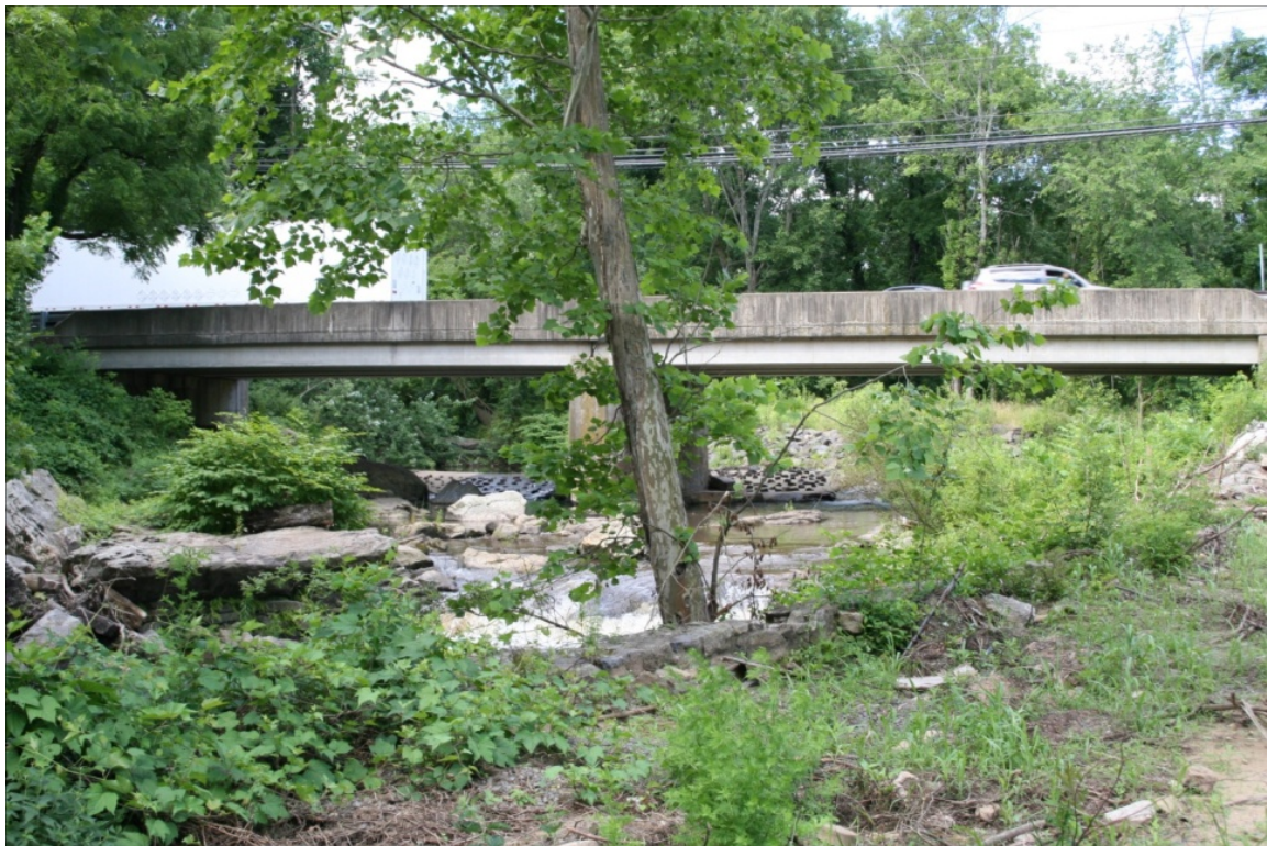
Buck Road Bridge, looking west
