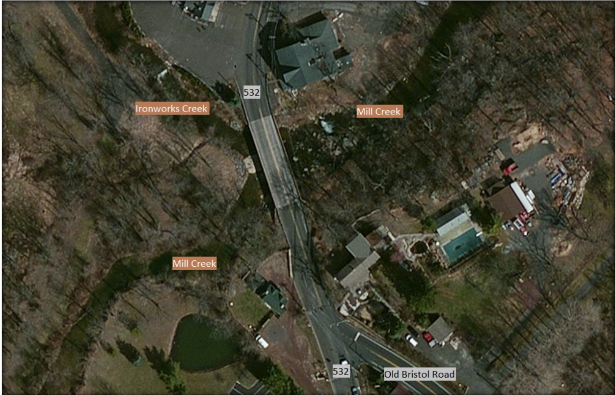
Figure 10: Overhead View of Mill Creek Bridge
