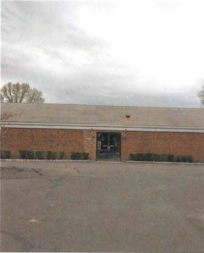
VIEW OF SWIM CLUB BUILDING
