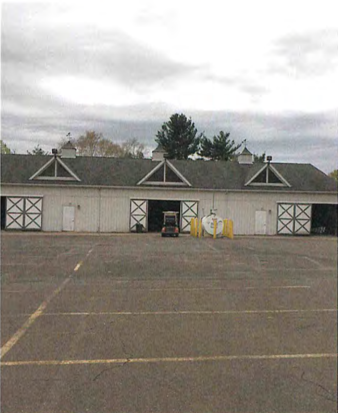
EXTERIOR OF CART STORAGE BUILDING
