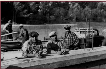
Circa 1942 photograph of workmen during the construction of the Churchville Reservoir Dam. Source: Courtesy of the Churchville Nature Center .
